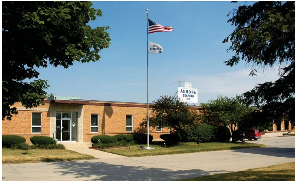
Aurora Bearing Company has been recognized worldwide for producing high quality and reliable products. Headquartered at 970 S. Lake Street, the company employs 200 people operating out of two facilities.
